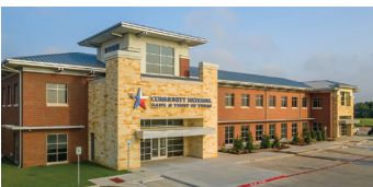
WAXAHACHIE BRANCH 1905 US Hwy 77 Waxahachie, TX 75165
